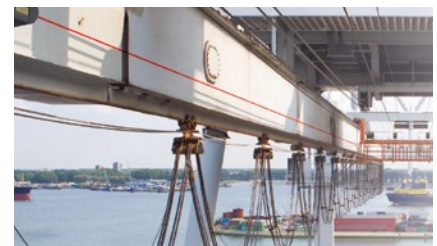
Position measurement on gantry cranes
